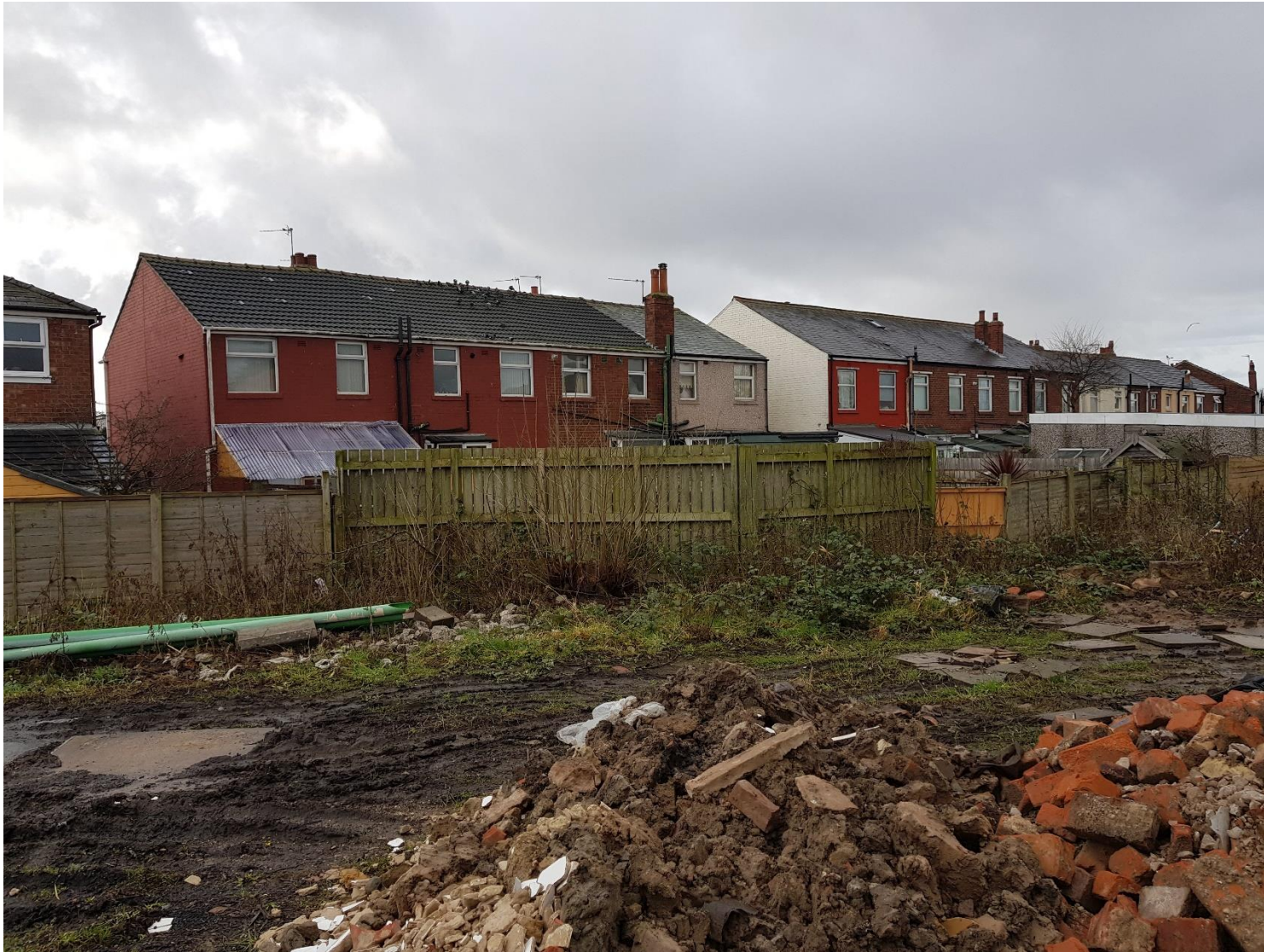
Properties on Cherry Tree Road backing on to the site
